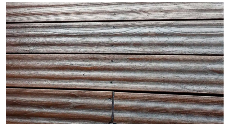
Renovated deck made from thermally treated ash after finishing with DeckFinish Color in dark brown.
