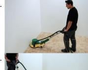
Use a single disc machine with a LOBASAND Perforated Pad P 100 alternatively a LOBASAND sanding net P100 and sand along the walls as close as possible to equalize the transition from edge sander to belt sander.
