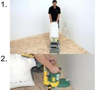
Sand the floor with a Belt Sander and a LOBASAND sanding belt P40. Depending on the type and pattern of the floor sand at a light angle or diagonal.
