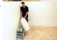
Perform the final cut with the belt sander and LOBASAND sanding belts P 120 into the direction of the wood. Drive as close as possible to the walls.
